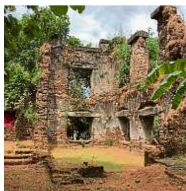
Remains of the Vypeenkotta Seminary built by the Portuguese, which lies adjacent to the Holy Cross Church
